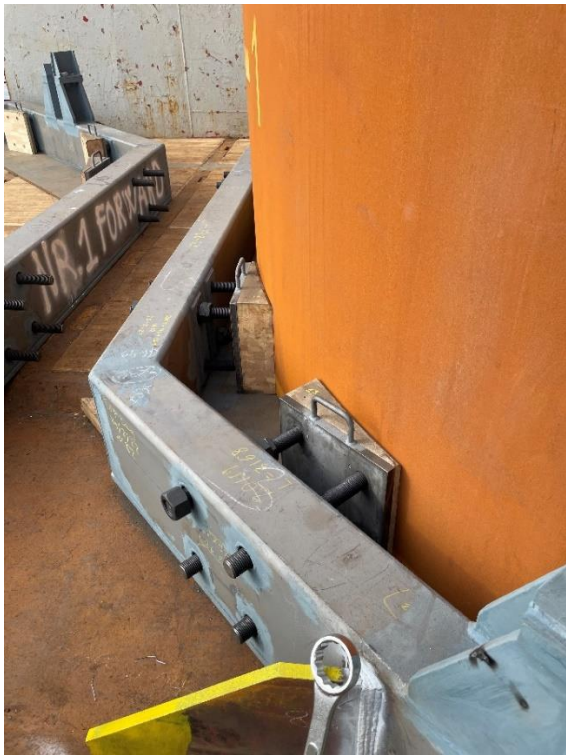
Semar effective seafastening at Hywind Tampen
