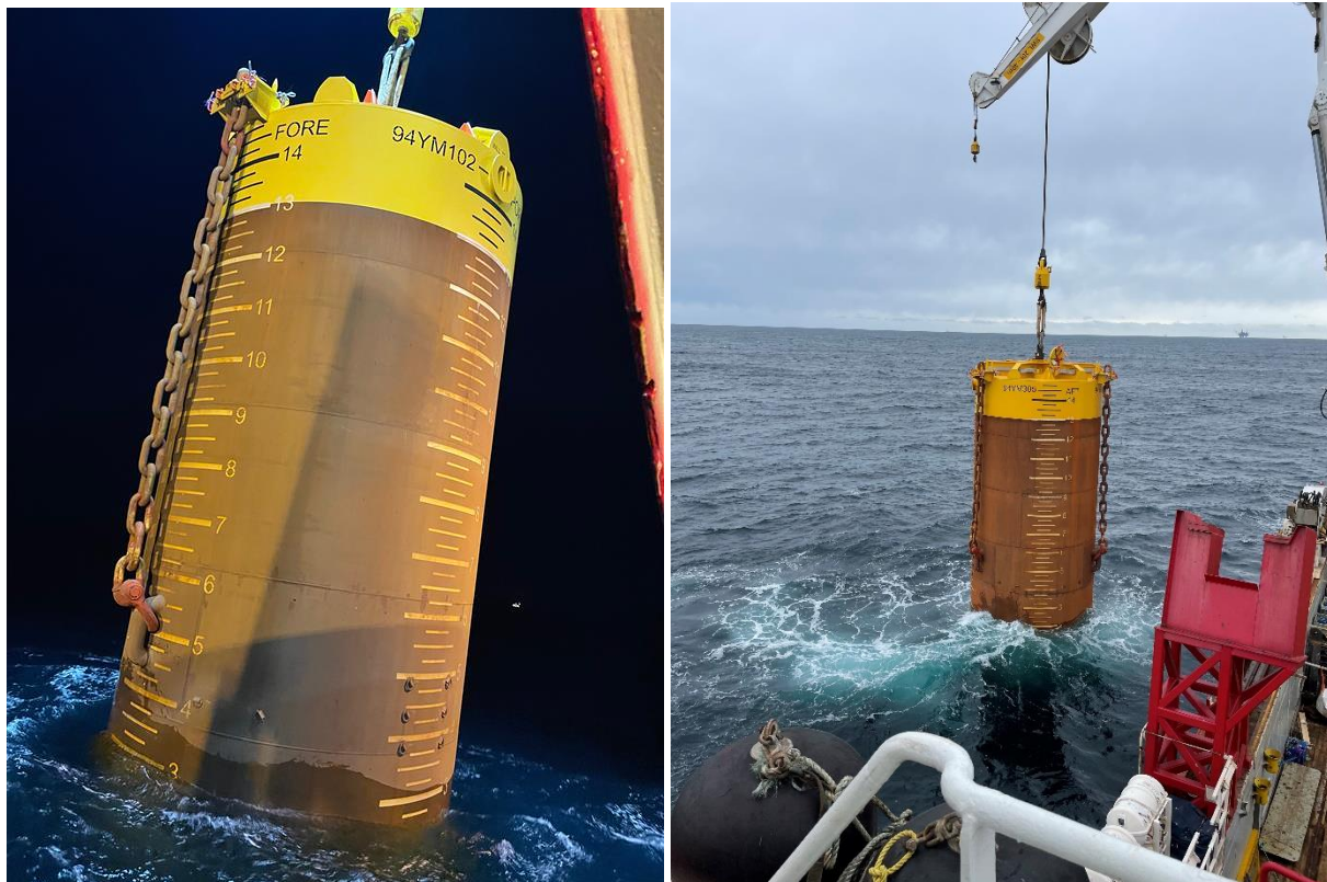
Lifting and installation operations at Hywind Tampen, Equinor.
