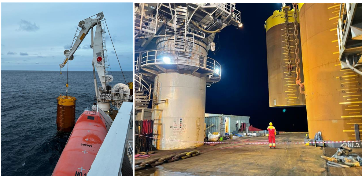
Pict.: SEMAR and DOF Subsea Installation of suction anchors at Hywind Tampen Q2-Q4-2022
